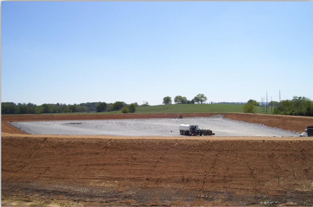
24 MG Earthen Inflow Holding Basin
