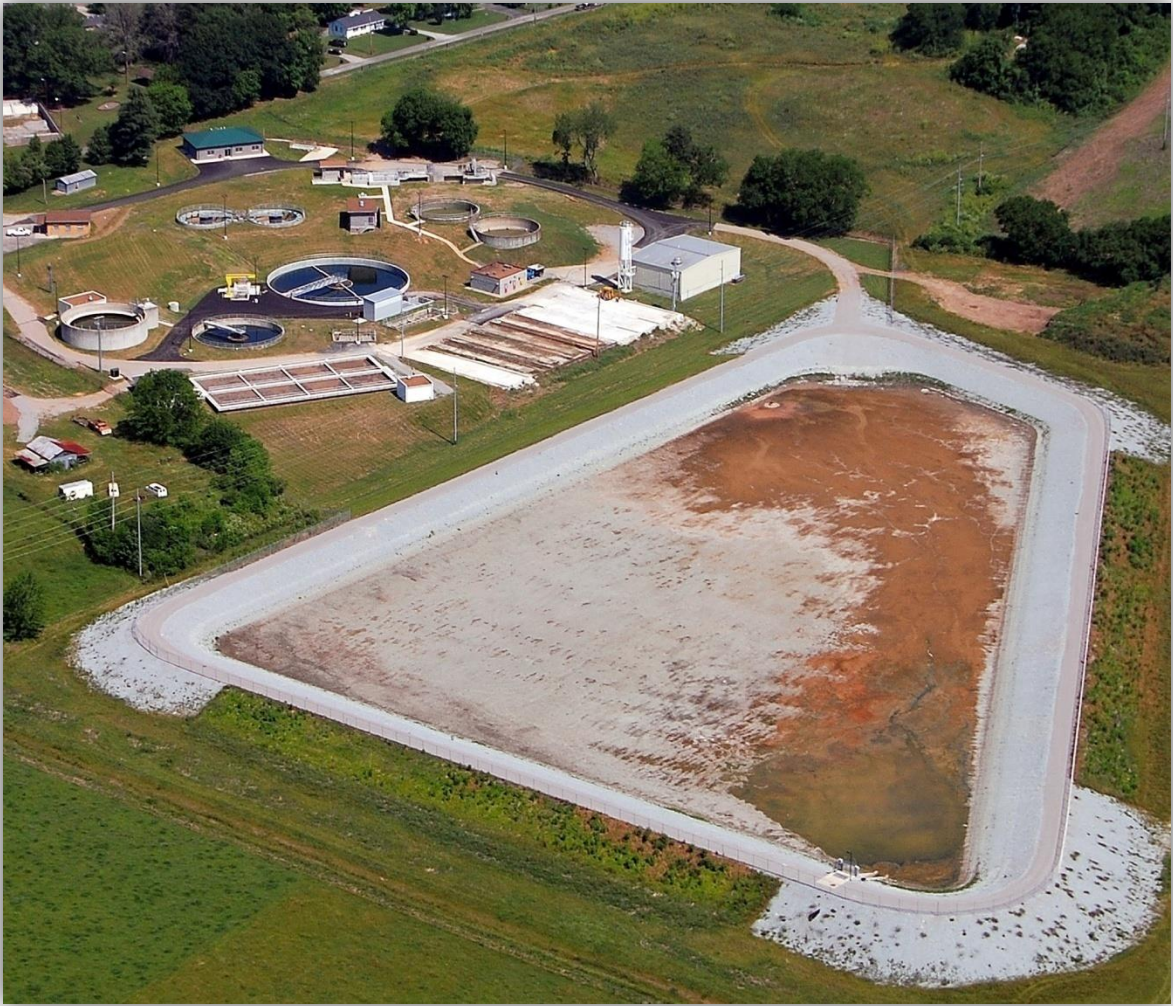
24 MG Inflow Holding Basin- Return Flow Pumping Station in Foreground
