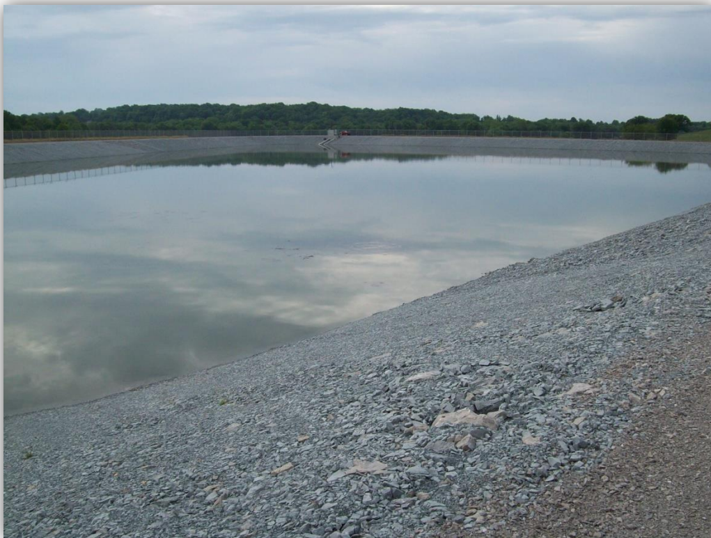
24 MG Inflow Holding Basin – Return Pumping Station in Background
