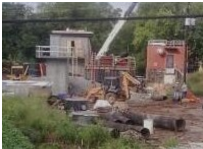
Construction of the 16.0 MGD Main SPS Pulaski, Tennessee
