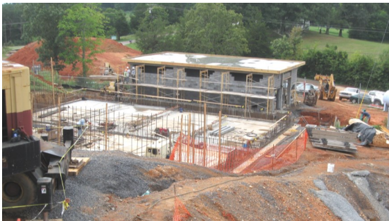
Pictured above in the background is High Service Pump Building and foreground is Clearwell Slab Water Treatment Plant – Dayton, Tennessee
