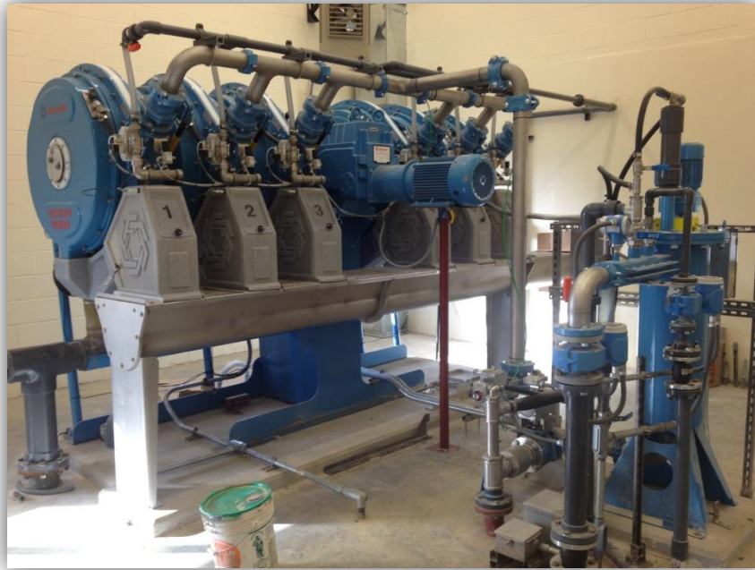
Rotary Style Sludge Press by Fournier Industries Lewisburg Wastewater Treatment Plant Lewisburg, Tennessee
